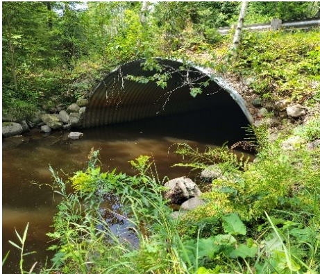
Bear Creek Rd. Culvert
