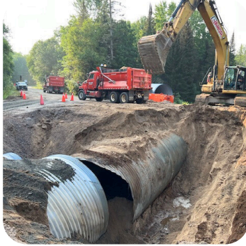
South River Rd Culvert Replacement
